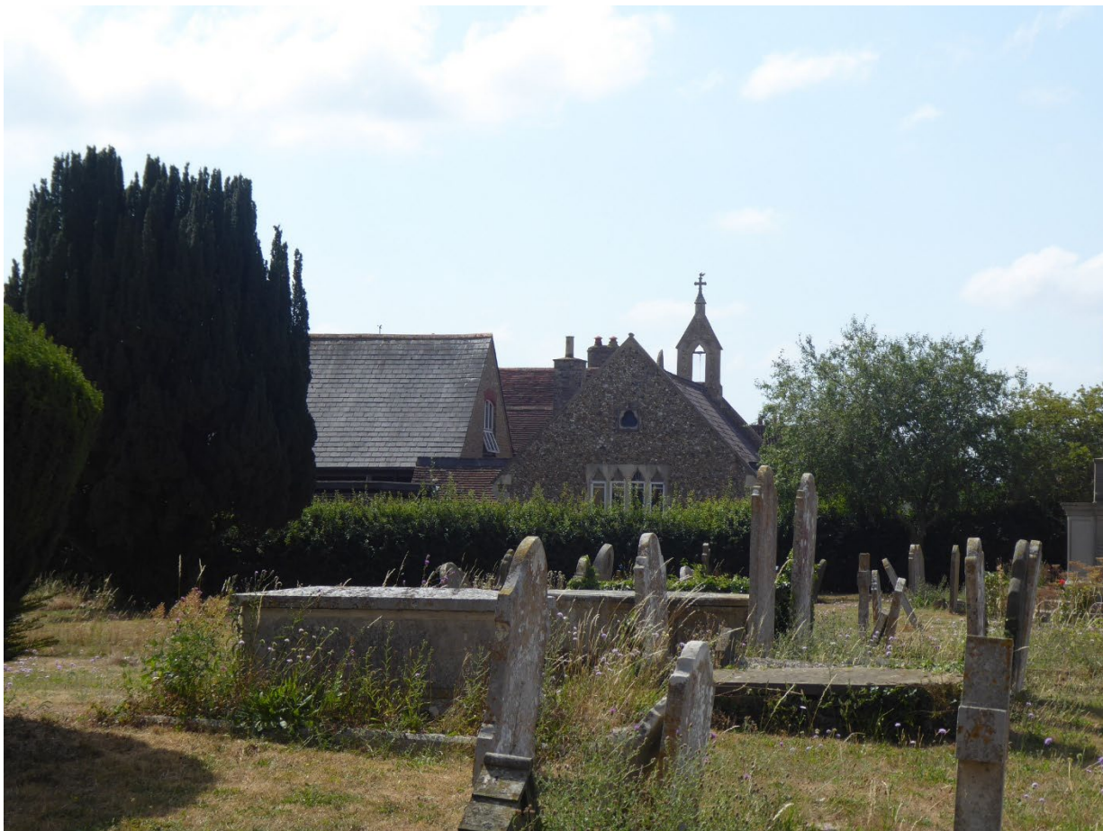
Figure 21 Rivenhall Church of England Primary School, viewed from the churchyard of the Church of St Mary and All Saints to the west.
