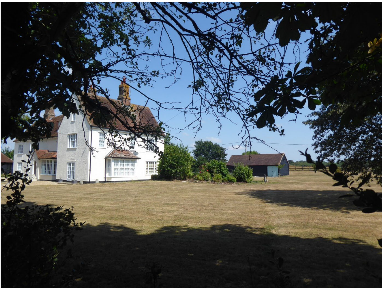
Figure 15 Clark's Farmhouse viewed from Cranes Lane to the south.
