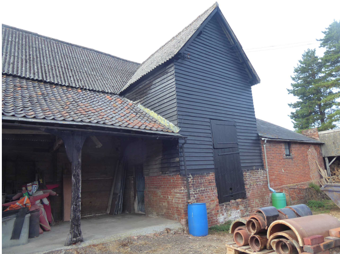
Figure 11 The Grade II listed Bentall's Barn
