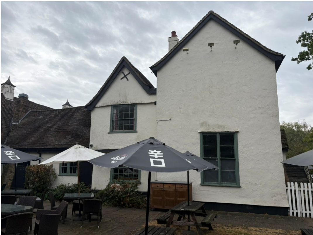
Figure 18 North eastern, side elevation of Fowlers Farm
