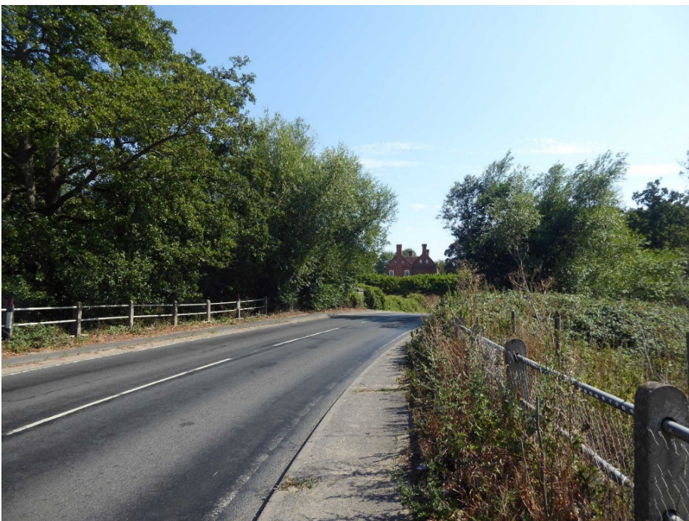
Figure 12 The Grade II* listed Bluebridge House, a prominent feature, looking south from Blue Bridge over the River Colne
