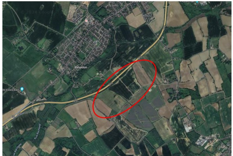
Land south of the A12, Kelvedon
