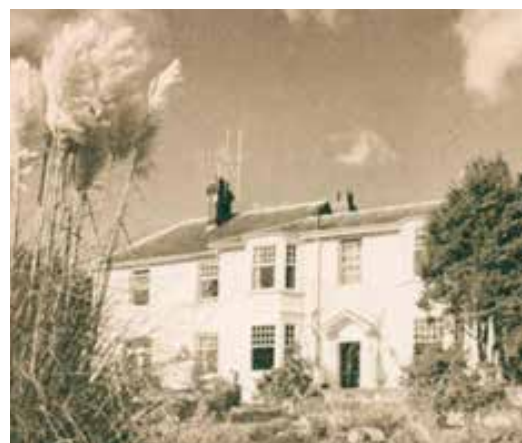
Figure 41 South elevation of the Hall (Wethersfield Local History Group)
