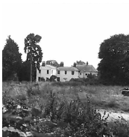
Figure 40 North elevation of the Hall 1984 (ECC)
