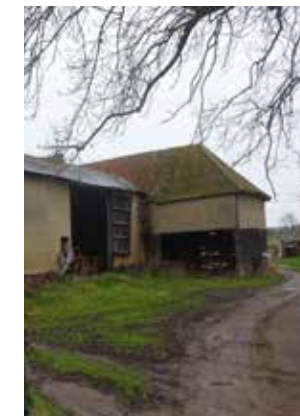
Figure 15 Weatherboarding and render, Russells Farm
