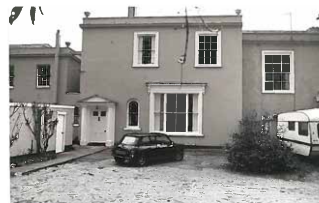
Figure 46 Separate driveways at Manor House [nd]
