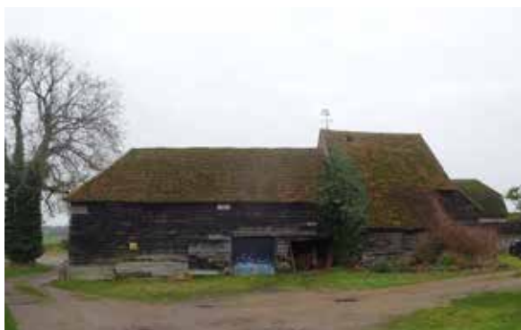
Figure 36 Listed barn and ancillary building, Russell's farm, Braintree Road
