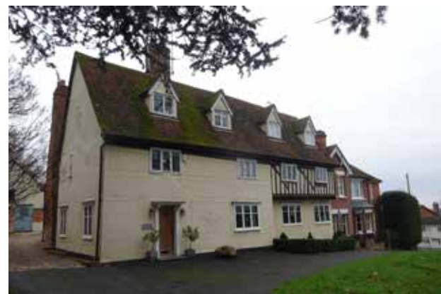
Figure 14 Example of pargetting, exposed timber framing and brick work at Ivanhoe House
