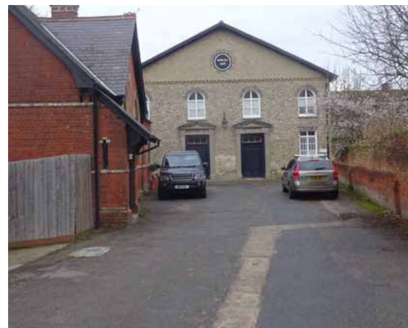
Figure 53 Hard Landscaping outside the United Reformed Church
