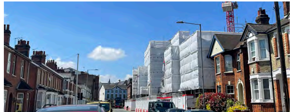
Figure 102 Manor Street development under construction, summer 2021
