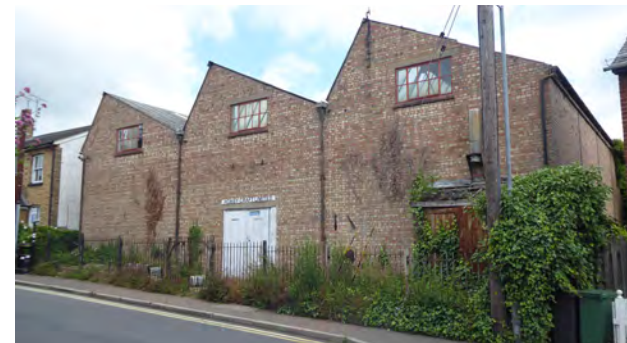
Figure 79 Saw-tooth roof, otley Road
