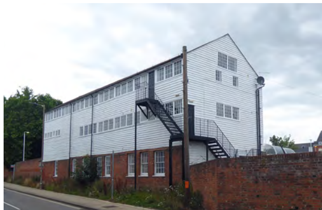
Figure 77 Pound End Mill, South Street, Grade II listed
