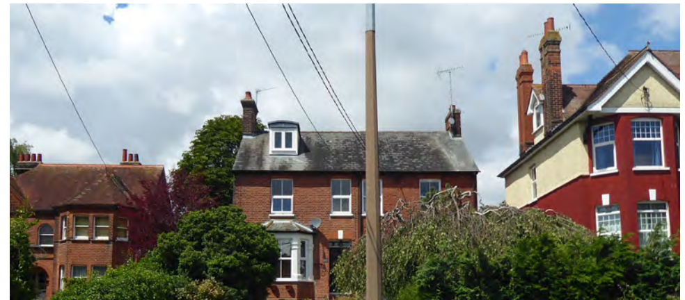
Figure 37 Examples of timber sash windows, brick, slate and painted render on London Road
