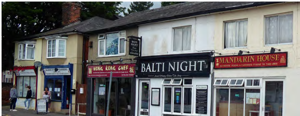
Figure 64 Shopfronts requiring improvement, Manor Street
