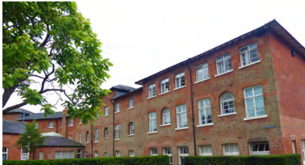
Figure 107 St Michael's Hospital, seen from the rear. The building is Grade II listed and now converted to flats
