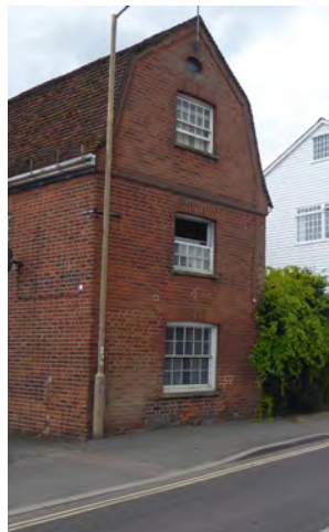
Figure 81 Red brick, South Street
