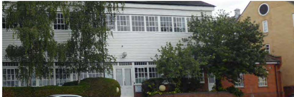
Figure 80 White painted weatherboarding on the Mill, with timber single glazed windows
