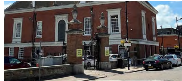
Figure 65 Walls and railings, Braintree Town Hall
