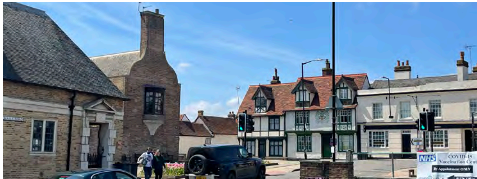
Figure 42 The junction of the High Street and South Street, by St Michael's Church
