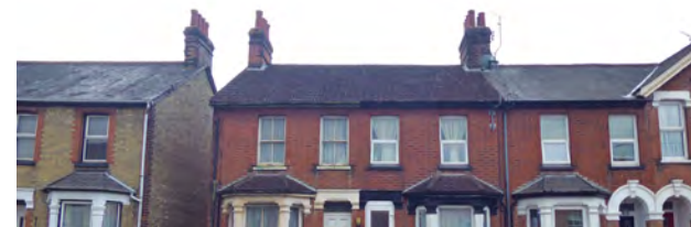
Figure 112 Example of timber sashes (second left) and uPVC replacements (right)
