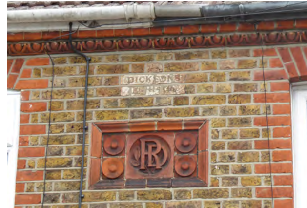
Figure 92 Example of decorative brickwork
