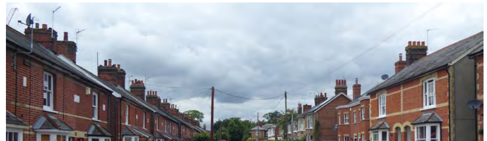
Figure 91 Roofs on Woodfield Road
