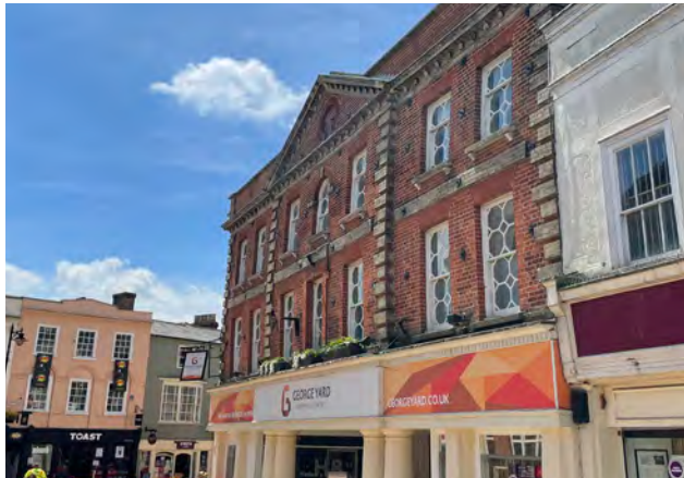
Figure 55 37-39 Bank Street, doubling as an entrance to George Yard
