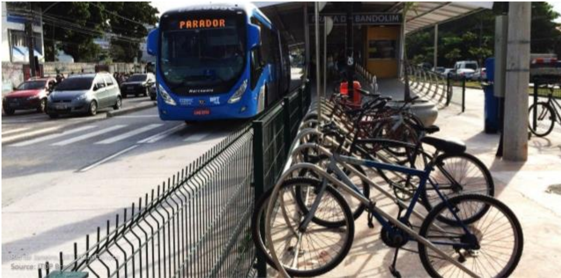
Figure 2-5: BRT station with cycling parking in Rio de Janeiro, Brazil Source: ITDP Brasil
