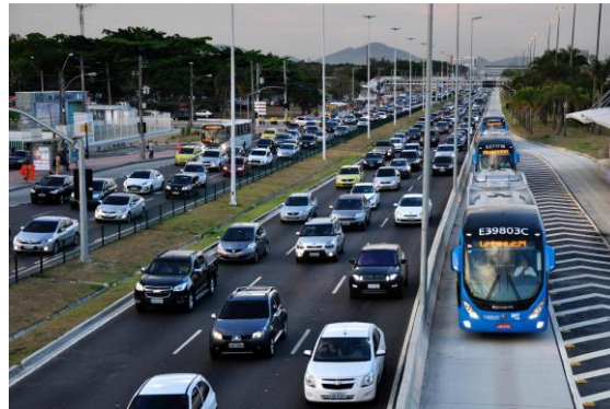
Figure 3-1: Route type 1: segregated – dedicated – Specially provided infrastructure for exclusive use of RTS in new roadway
