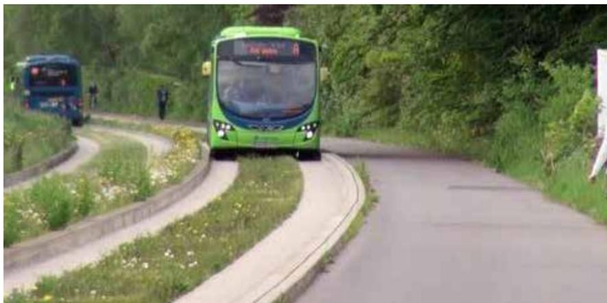
Cambridge Guided Busway - an example of the type of solution that could be implemented on the Flich line. Operational since 2011 it runs for 25km and connects Cambridge to Huntingdon (60min) and Trumpington (15min). It runs at a 7 minute frequency and reaches speeds of 90kph. Image Source: Google
