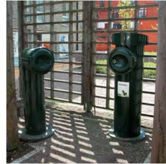
Image 79 Domestic waste chutes to underground storage, Malmö
