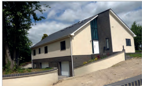
New residence on Lucking Street (north)
