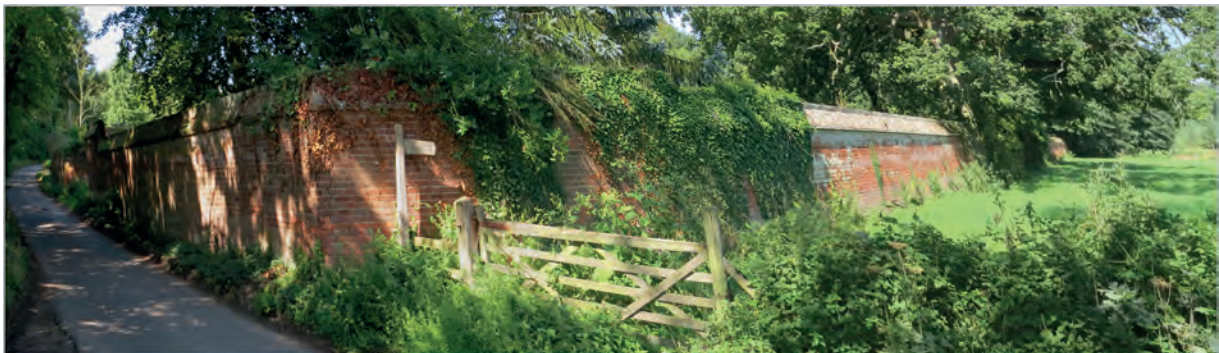
The lower section of St Mary's wall
