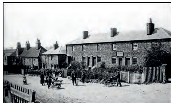
Stone Cottages in Church Street
