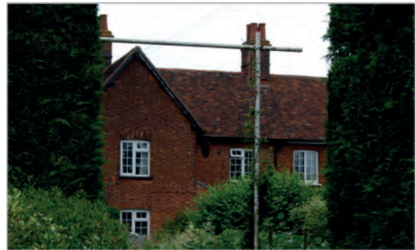
Style of brick construction cottages
