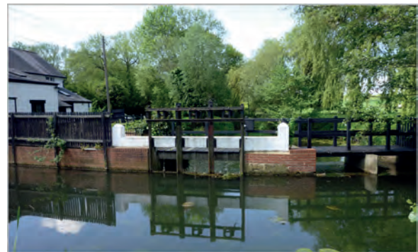
River Colne passing over the Hulls Mill weir
