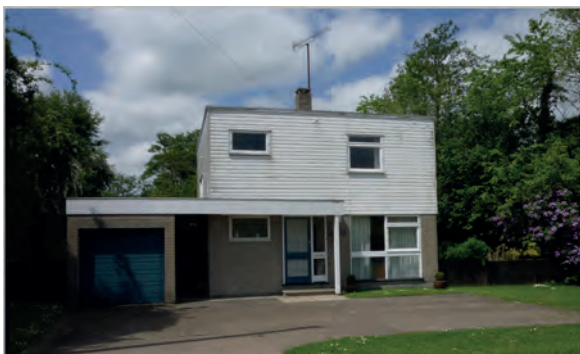
The former village nurse's house
