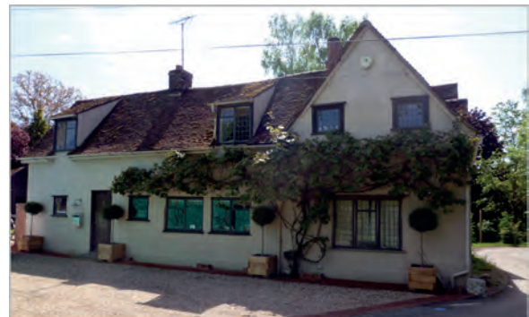
16 th century painted plaster rendered dwelling
