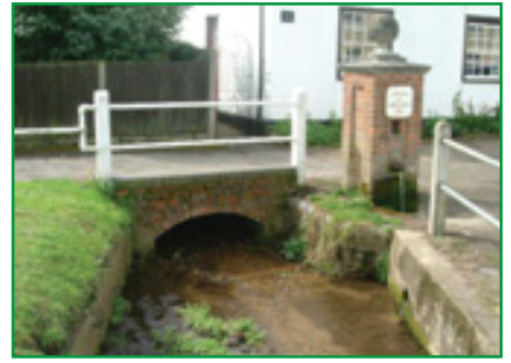
▲ The Fountain erected by Henry Smith 1860
