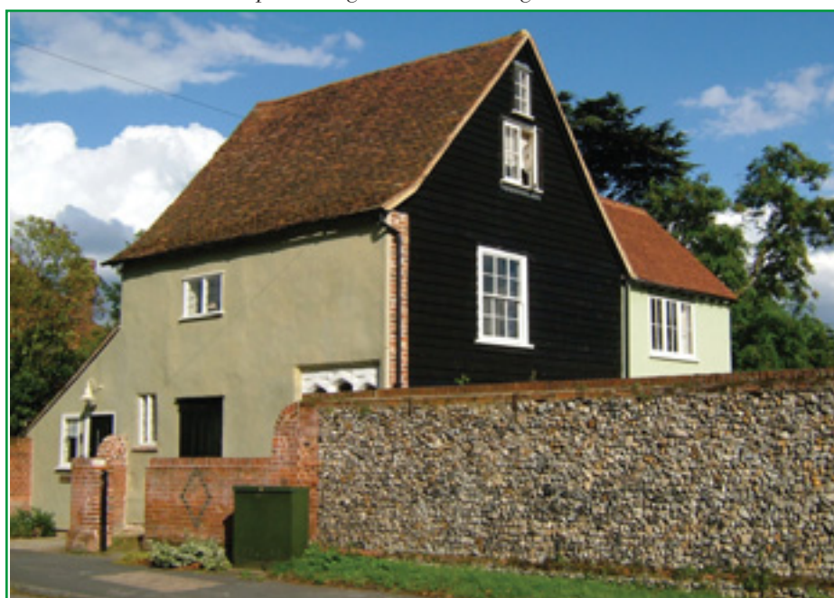
▼ Chapel Cottage renovated using lime mortar
