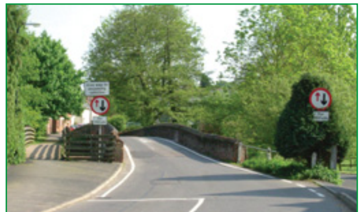
▼ Bridge over the River Pant
