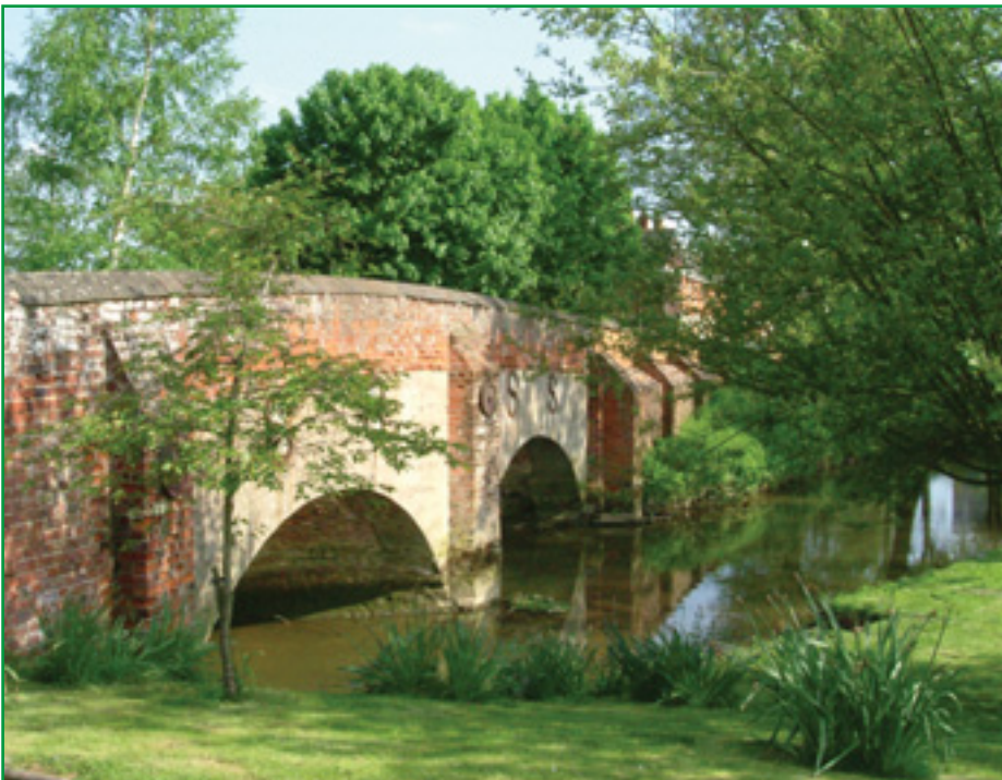
▼ Bridge over the river Pant
