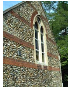
The Gothic style window set into flint & brick wall.
