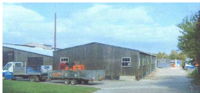
Farm buildings now used as business units.
