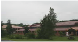
Purpose built units in a sympathetic setting on the Business Park
